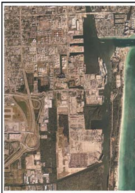
Aerial View of Port Everglades
